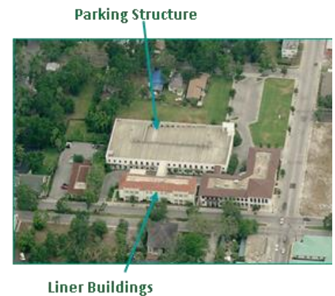
Figure 18. Detached Liner Building
